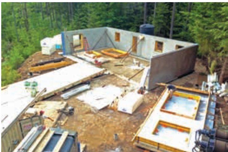
Damon Gray notes that highly energy efficient building with panels costs no more than standard building
