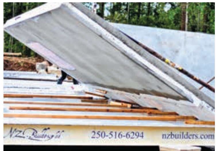
Building with concrete sandwich panels is still unique in residential construction
